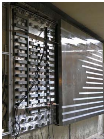
The workings of the LEDs and drivers, and the installing into the underpass
