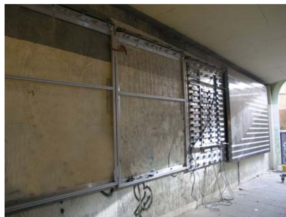
The workings of the LEDs and drivers, and the installing into the underpass
